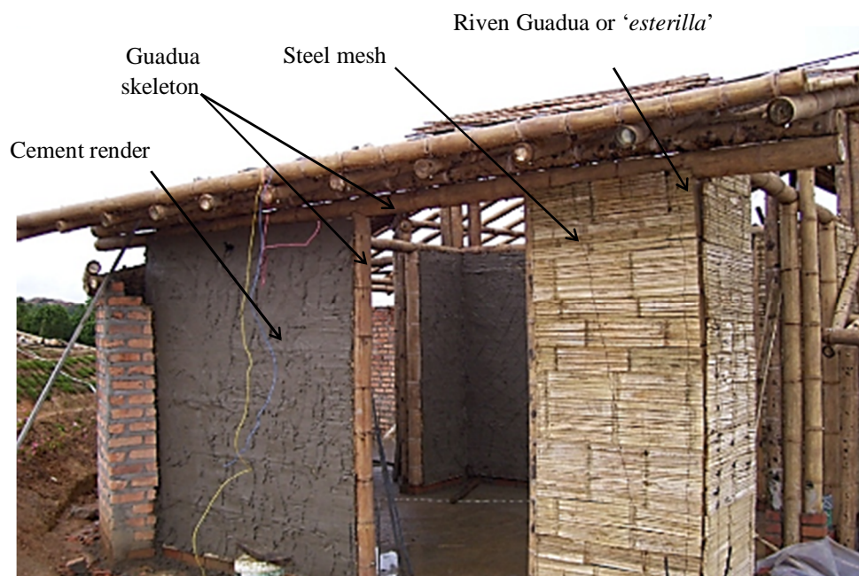
Figure 1. Plastered cane wall-framing system
