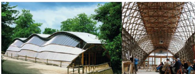
Figure 2.6: Weald & Downland gridshell; exterior with triple hour-glass shape; interior view (from Architect's Journal Building Library)
