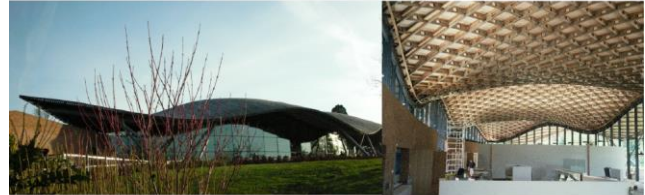
Figure 2.7: Savill Garden gridshell; exterior with corrugated vault shape on slanted steel supports; interior view (images – Richard Harris)
