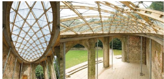
Figure 2.8: Chiddingstone gridshell; interior view; detail of grid layout showing two layers, nodal connector and shear blocks (from [7])
