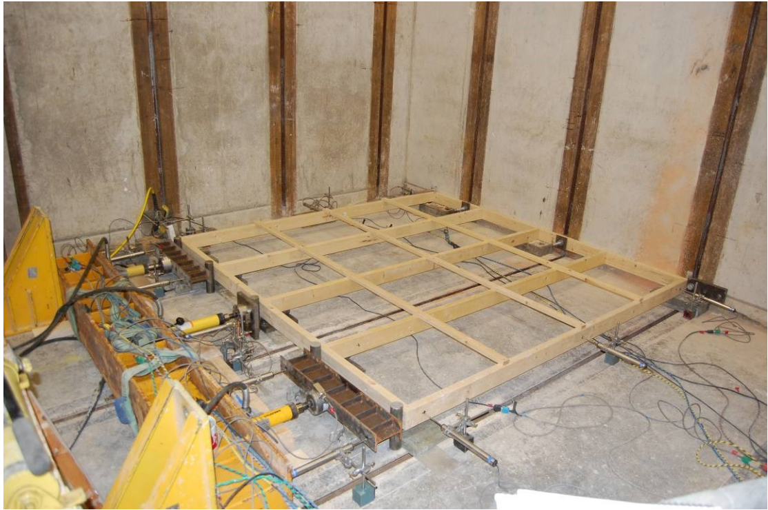
Figure 4 Wall R3 in test rig
