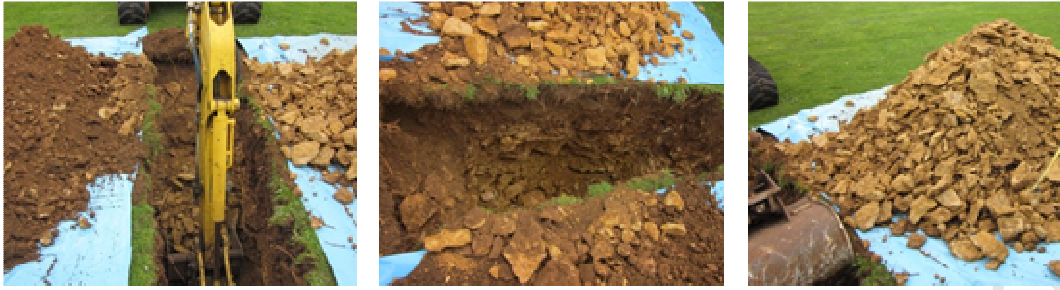
Figure 1: Frost-shattered oolitic limestone (FSOL) unearthed during the site investigation
