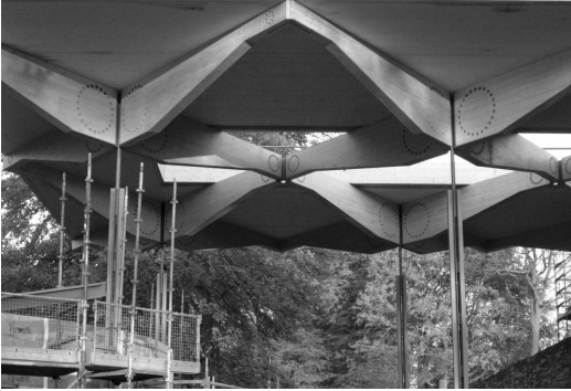
Figure 4: The roof construction over the entrance lobby (Image copyright: Buro Happold)
