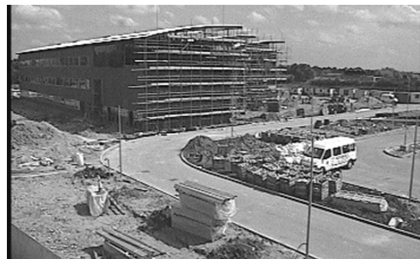
Figure 6. Web Camera Image of Microsoft Research Laboratory under construction, 22nd June 2001
