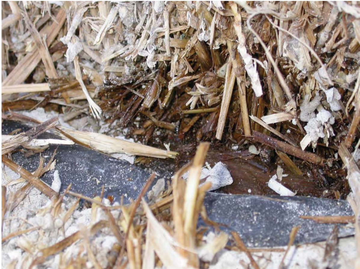
Figure 2: Straw behind a rendered wall kept in high moisture conditions
