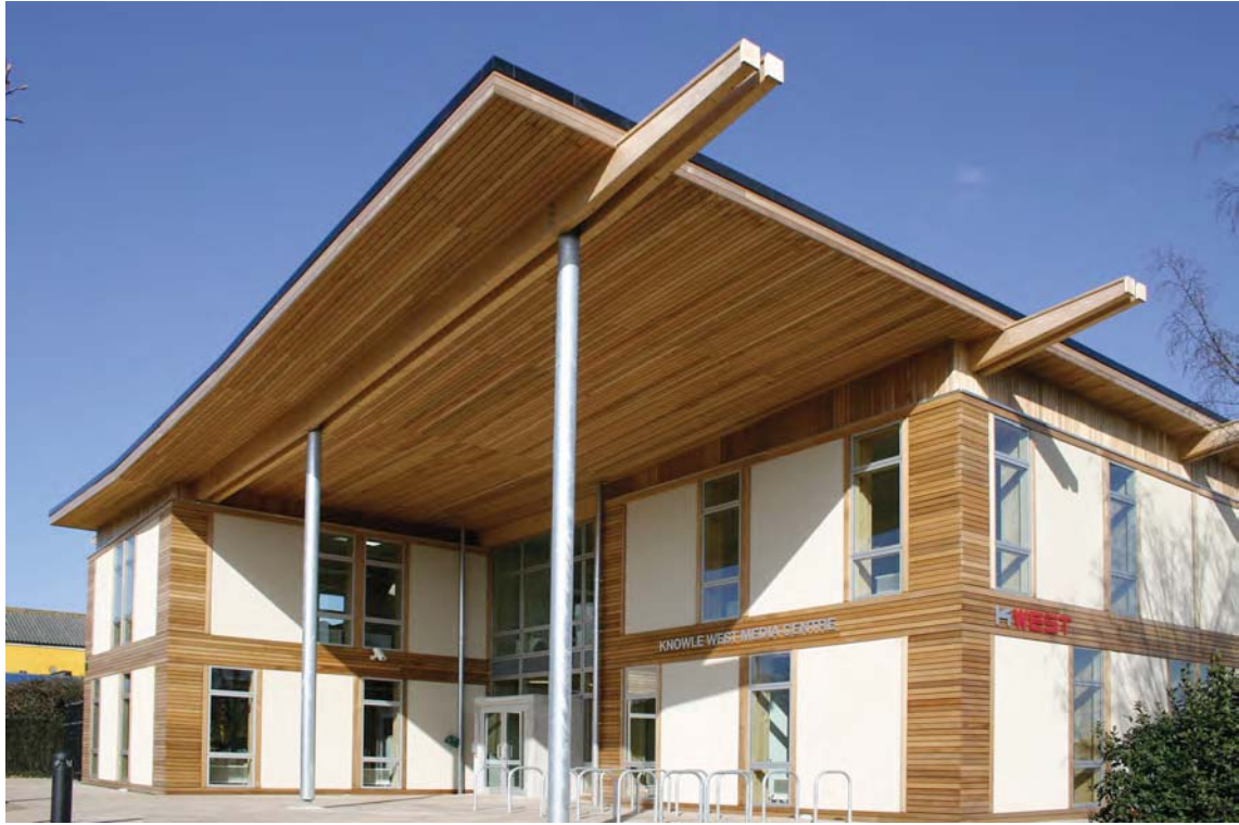
Figure 1: Media centre in Bristol constructed using ModCell pre-fabricated straw bale panels
