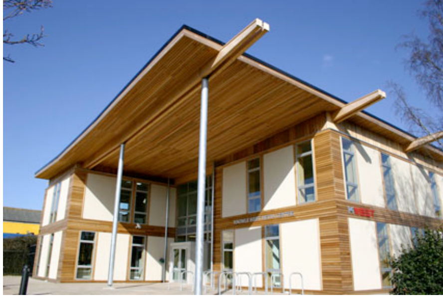
Figure 2: Media Centre in Bristol constructed from straw bales
