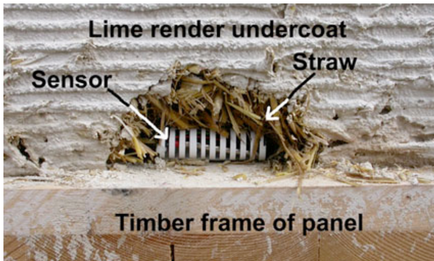
Figure 3: Sensor inserted just below the external render (prior to final rendering)
