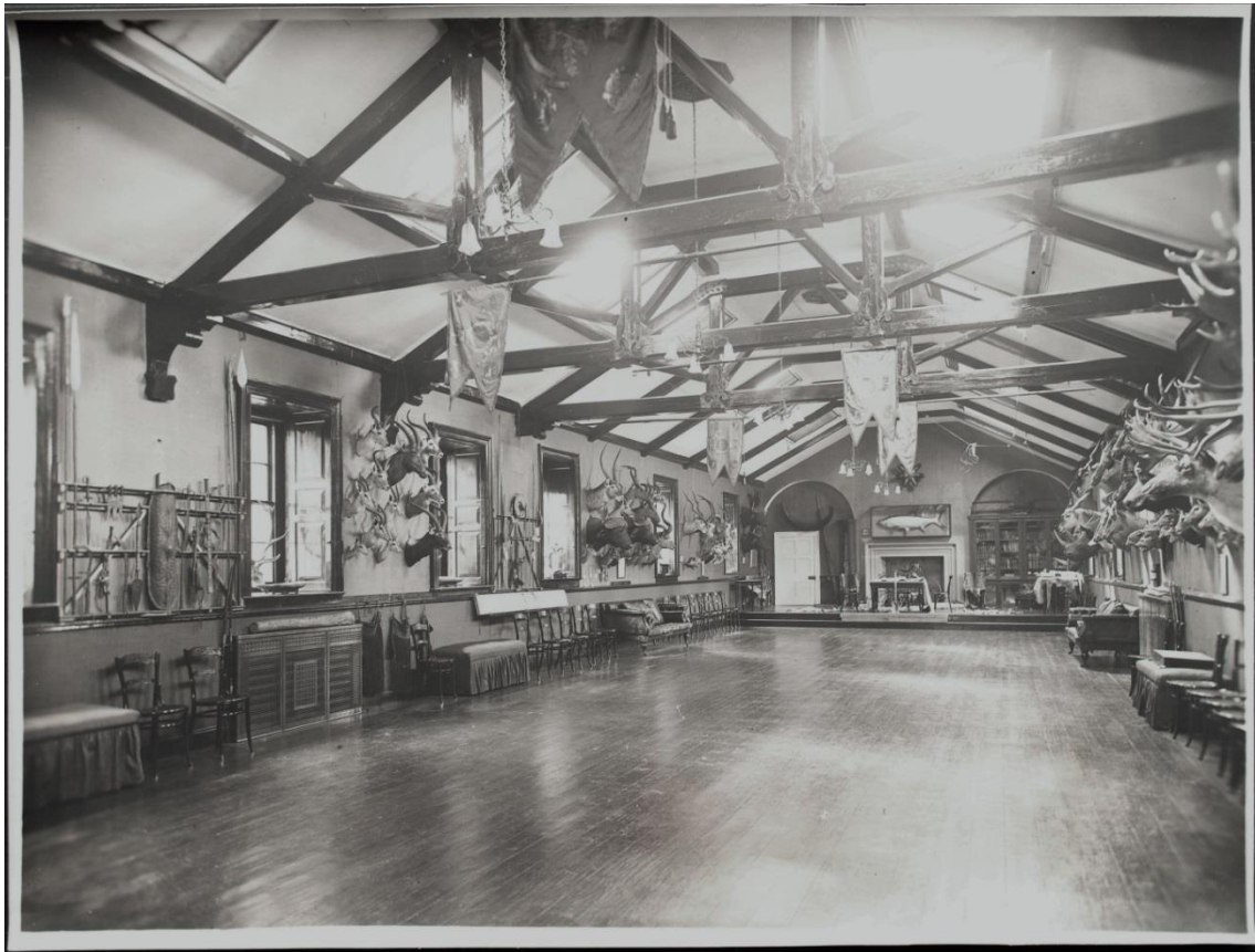
Figure 87: Tatton Park Tenants Hall pre 1935
