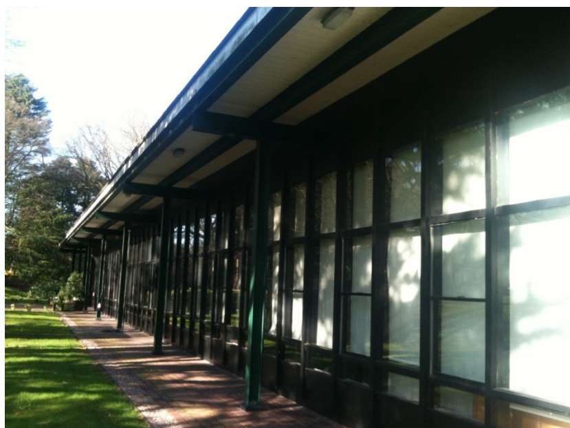
Figure 5. Cuerden Pavilion, Cuerden Hall, Lancashire, designed by Robert Matthew Johnson Marshall, 1971 (photo by Victoria Jolley).
