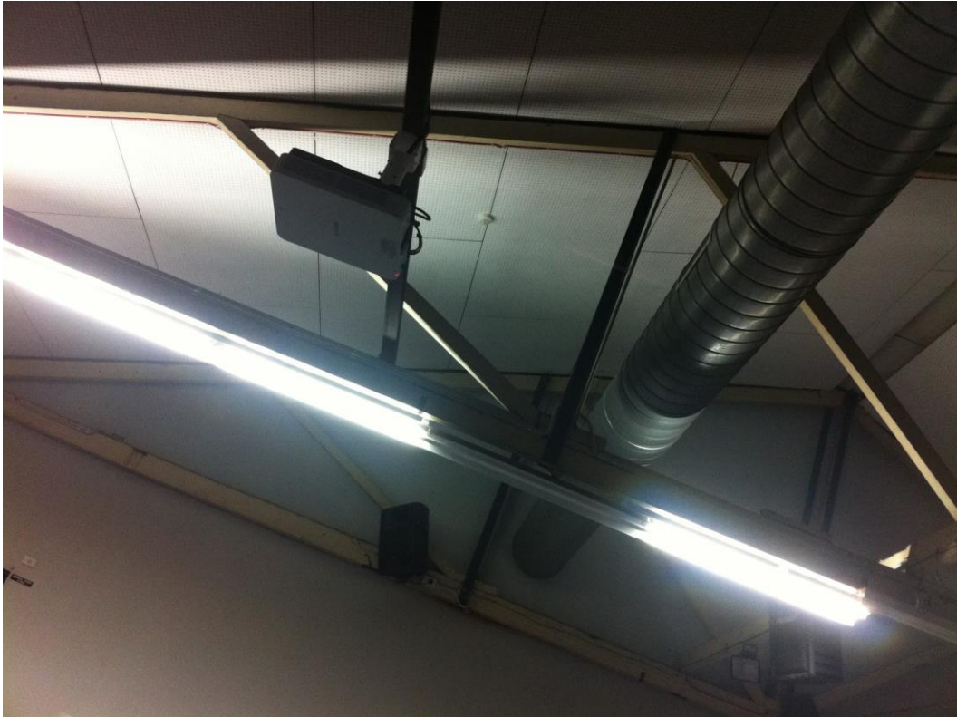
Figure 4: Victorian College of the Arts Art Auditorium ceiling
