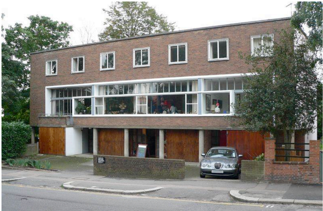
Figure 1: 2 Willow Road, London. Source: http://en.wikipedia.org/wiki/File:1_2_3_Willow_Road_Hampstead_London_20050924.JPG
