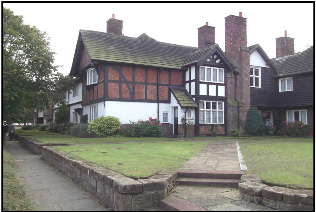
Two views of 'mock-Tudor' houses at Port Sunlight. These and the following photographs illustrate how Mawson's ideas may have been influenced by designs at Port Sunlight.
