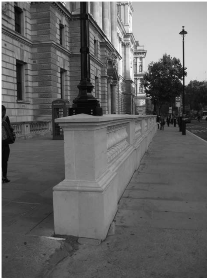
Figure 3. Security Balustrade Along Whitehall, London (January 2009)
