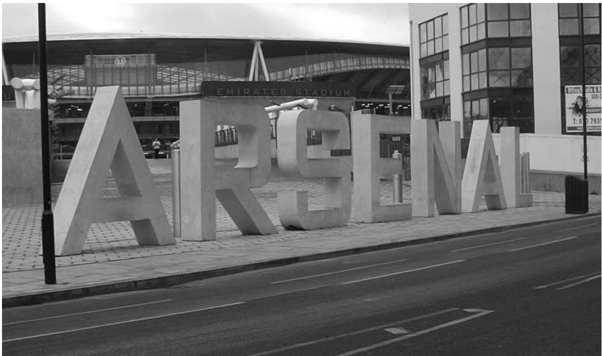
Figure 5. 'ARSENAL' – Ornamental Security Façade for the Emirates Stadium (July 2003)
