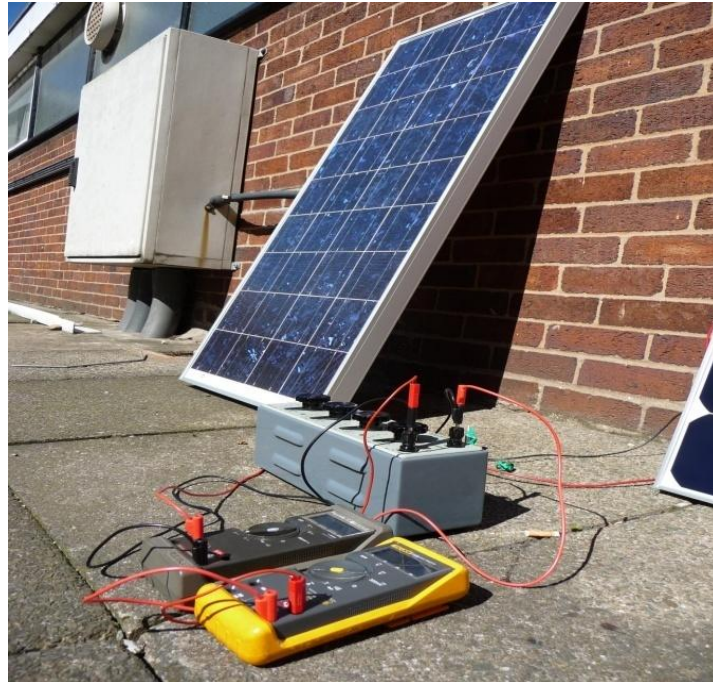
Figure 6.6 - The experimental test rig
