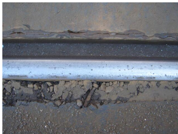
Figure 5.31 Photographs of damaged polymer. Polymer protects the rail from degradation such as rust and helps dampen noise and ground vibration.
