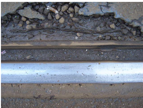
Figure 5.31 Photographs of damaged polymer. Polymer protects the rail from degradation such as rust and helps dampen noise and ground vibration.
