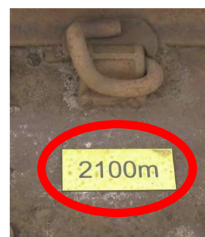
Figure 5.28 A photograph of a distance marker on Staton Bonna bi-block. A distance marker shows the distance from a known datum
