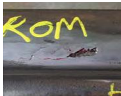
Figure 5.45 A Photograph of rail cracking caused by RCF development over time.
