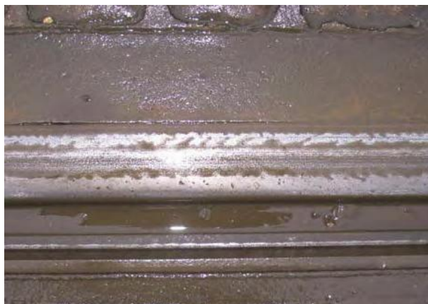
Figure 5.30 A photograph and graphical model of grooved rail. This is used in urban environments where vehicle and pedestrian traffic intersects with the track.
