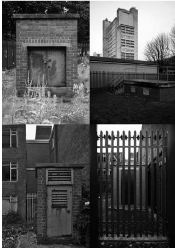
Figure 5. [image top left] The small surface building at the top of cable tunnel as originally constructed, Lockton Close, Ardwick, Manchester (Source: Courtesy of George Coney). [top right] The same location after being rebuilt and secured in 2005 (Source: Richard Brook). [lower left] The small surface building at the top on cable tunnel, Islington Street, Salford (Source: Courtesy of George Coney). [lower right] Additional security fencing installed around Islington Street access point. (Source: Richard Brook).
