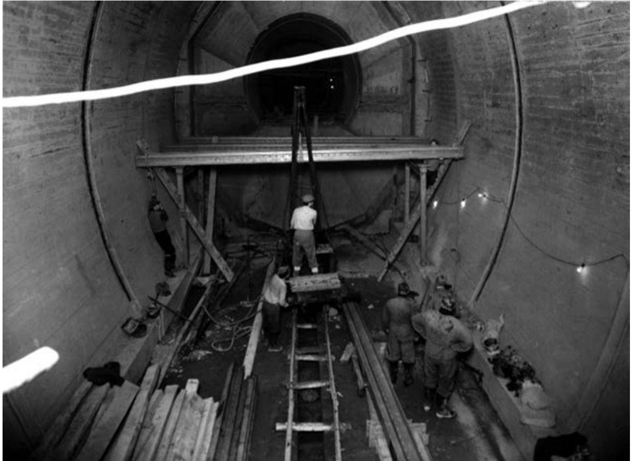
Figure 8. Original photograph documenting the construction of the GUTE , dated March 1956. The scale of the main equipment tunnel is evident and this was eventually subdivided to create two working levels. The formwork for concreting in the main tunnels was steel, but the connecting points between the tunnels were made by specialist joiners from timber. (Source: Photograph by tunnel engineer Patrick Gough. Courtesy of George Coney.)
