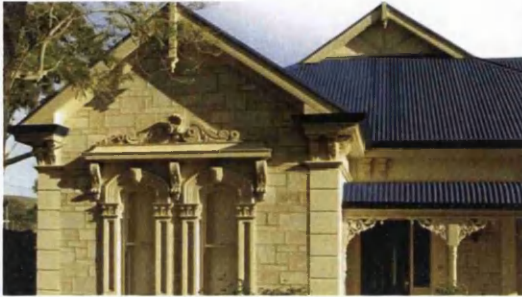
(c) Corrugated roof and walls ( http://www.gulfcoastsupply.com )
