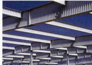
(b) Beams with corrugated web ( https://www.hera.org.nz )
