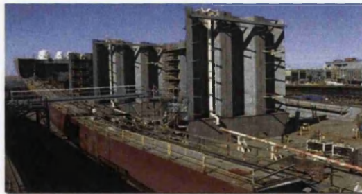
(g) Corrugated bulkheads in ships ( http://www.nassco.com )
