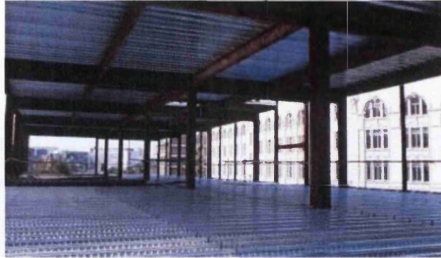
Figure 2.12: Composite floor structure (CP&P 2002)
