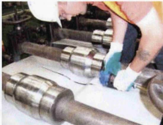
Figure 6.4: Cutting using a pneumatic cutter.
