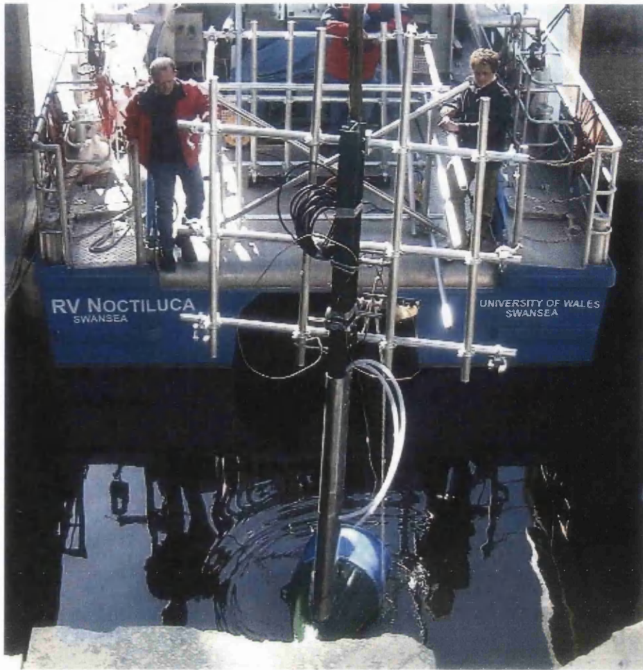
Figure 3.19 - Turbine being installed by marina crane
