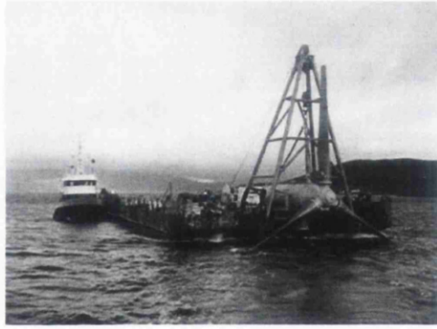
Figure 2.07 - Hammerfest Strom device being transported to the installation site.
