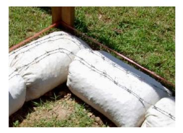
**Figure 5:** Barbed wire layour. Source: Geiger, O. (2015, September). Earthbag Building Guide (Abridged and Adapted for Builders). Special Edition by Osho Tapoban Publications.
