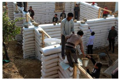
Figure 12: Good Earth Nepal construction of an Earthbag school, Makwanpur, Nepal
