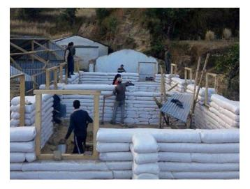
Figure 3: Earthbag Construction, Makwanpur, Nepal
