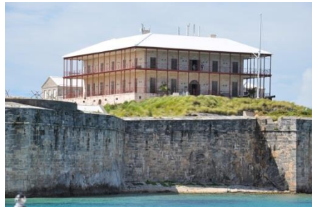
Figura 18. La Commissioner's House, Royal Naval Dockyard. [48]
