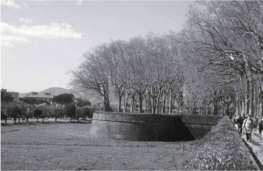
Fig. 6.6. The old city walls of Lucca, in Italy, had trees planted on them to help dry out the earth fill and make them stronger fortifications. Their defensive purpose has long ceased to exist, so that they make a very attractive, shady walk right around the old city ( photo: S. Bell )
