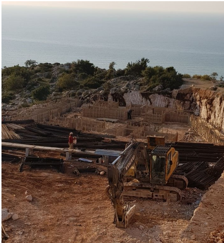
Figure 3 - Sama Residence, under construction
