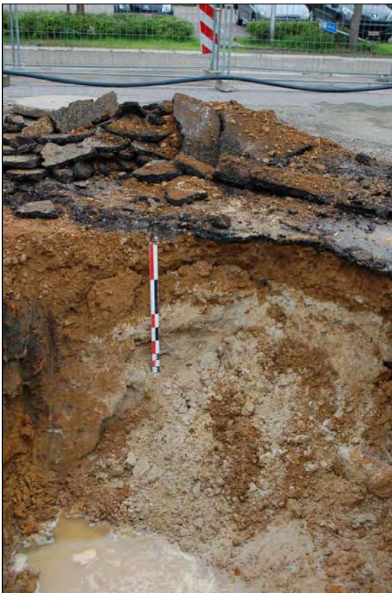
Fig. 11: Ingestort profiel in PP5.
