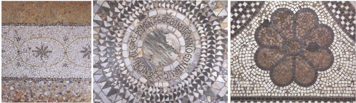
Figure 2 Different types of Venetian terrazzo flooring finish
