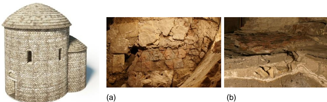
Figure 3 Rotunda 3D structure (Church of St. Wenceslas) at left hand side, (a) Brick tile floor (b) Cross-section of floor layers.
