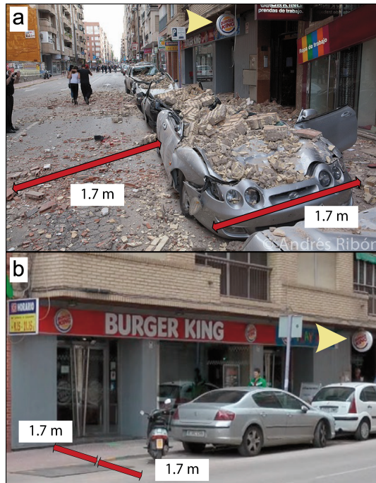
Figure 4. An example of how maximum impact distance was calculated. The yellow arrow shows a common reference point for the two pictures (the round restaurant logo). Image (a) was taken a few hours after the earthquake. Image (b) was taken 4 days after the earthquake. Photographs: (a) Andrés Ribón and (b) Marc Bertran Rojo.
