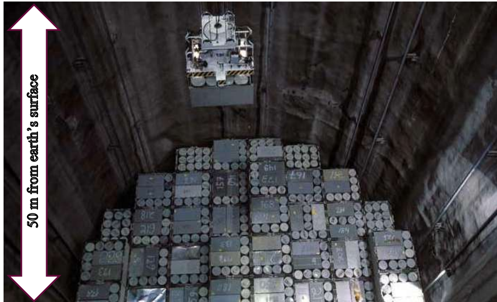
Figure 2.3: Mouth view of the geological repository at TVO, Finland for LLW (Image credit: STUK's 2014 report on the safety of spent fuel management.)
