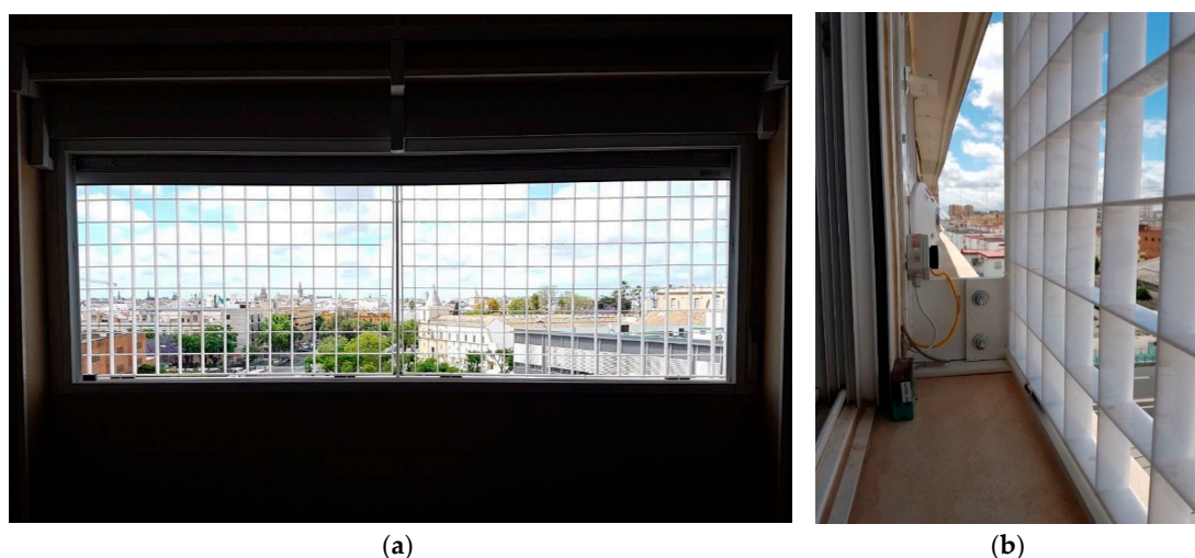
Figure 4. Egg-crate device designed: (a) indoor view; (b) outdoor view.
