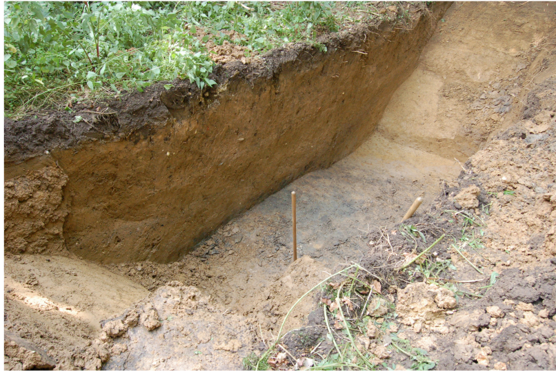
12 Trench 41: section during cleaning prior to collapse
