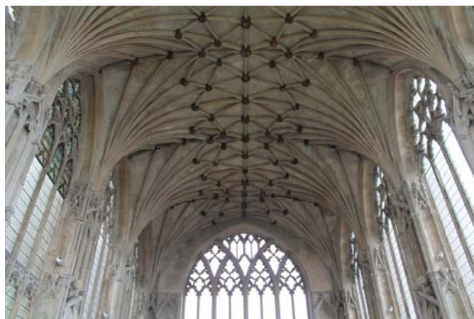
Fig. 1. Lierne vaults in the Lady Chapel at Ely cathedral.
