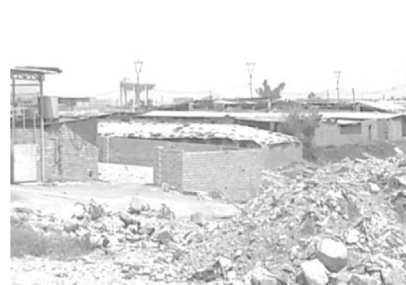
Informally self-built houses
