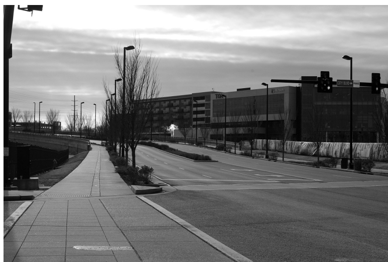
Figures 13a and b. A Complete Street intersecting Charlotte Avenue includes integrated bicycle paths, pedestrian walkways, trees planted as a safety barrier, and a street for cars and buses. An adjacent street leading into One City is marked as 'Private' to indicate the developing neighbourhood as a place of exclusive commerce.
