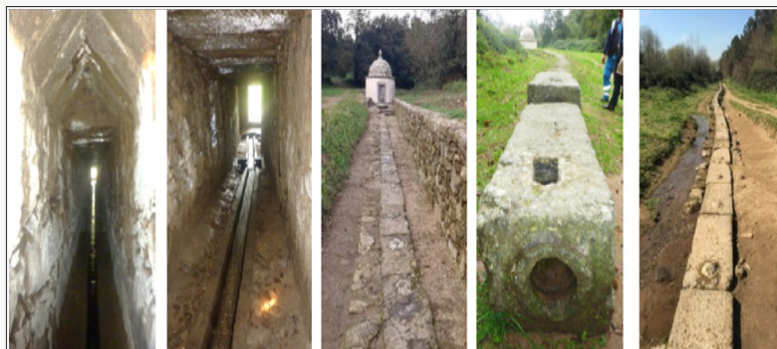
Figure 7: Details of the underground branched galleries and the stone aqueduct channel of Sete Fontes water supply system (Braga, 18th century).
