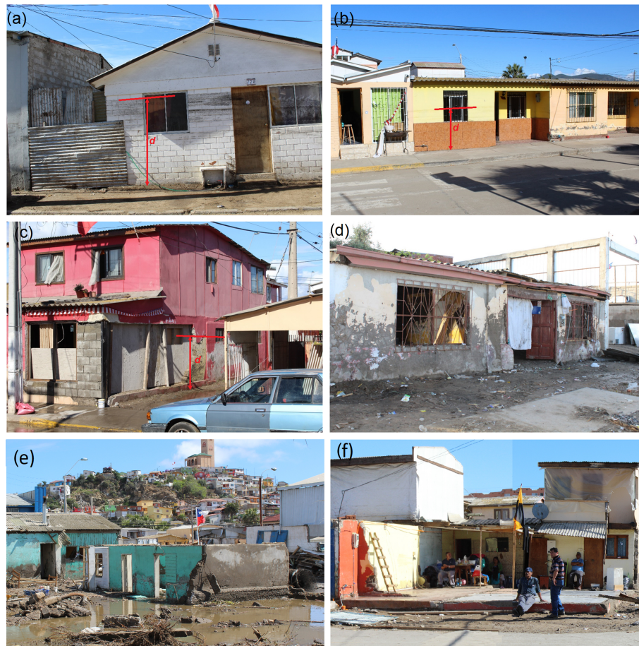
Figure 2. Photographs of structures undamaged and masonry houses damaged by the 16 September 2015 tsunami in the Coquimbo area. The red letter d indicates the observed tsunami inundation depth. All photos were taken on 22 September 2015.
