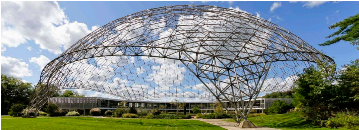
Figure 1. Geodesic spatial frame approximating a quadric surface: American Society for Metals International Headquarters and Geodesic Dome, at the Materials Park campus in Russell Township, Ohio, United States (Source: https://theredlist.com/wiki-2-19-879-605-285216-view-buckminster-fuller-richard-profile--1.html ).
