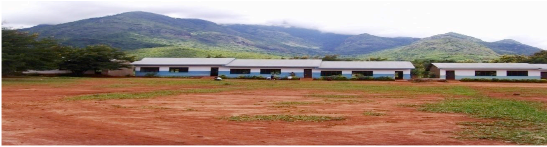
Figure 5.2 (a) Photograph of the part of Lupanga Secondary School
