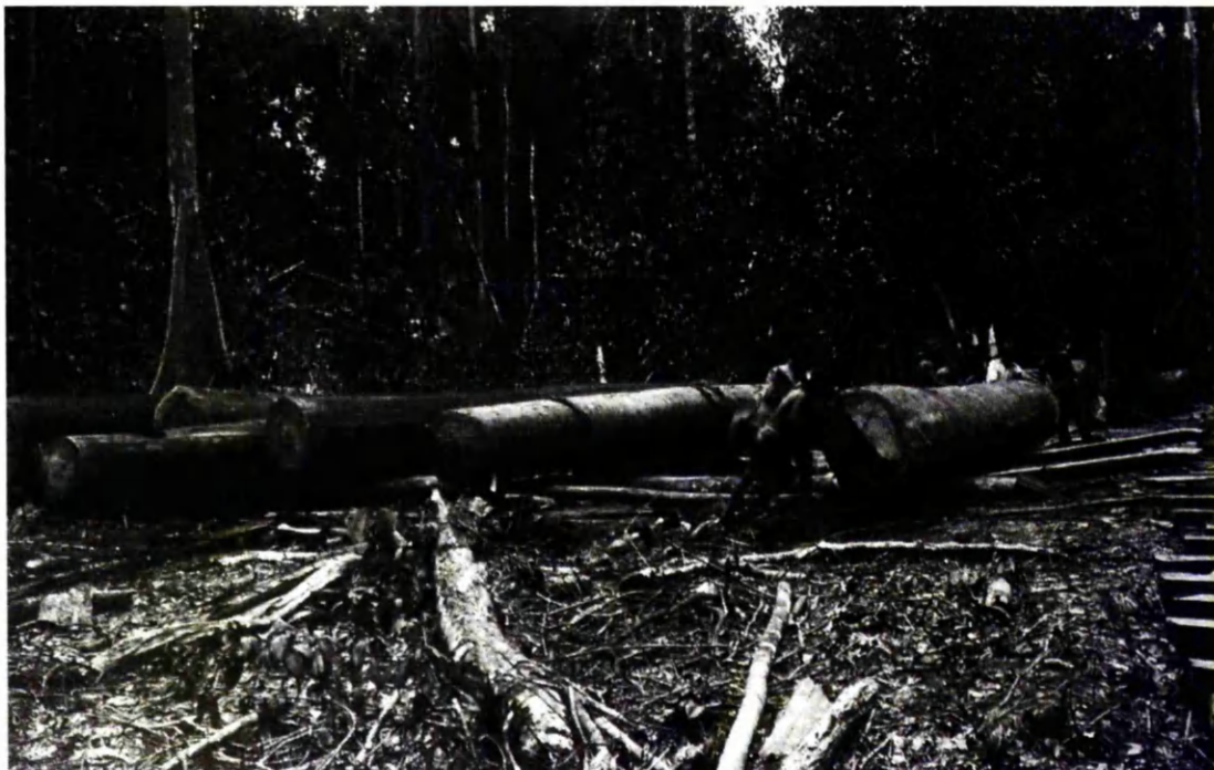
5. Labourers working on timber camp
