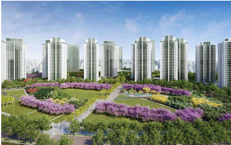
Figure 73. View of 1st Phase of Agua Branca ‘Reserva Manaca’. Source: Tecnisa, 2012.
