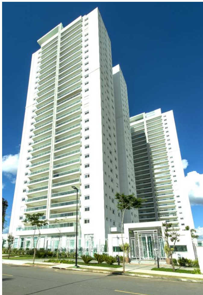
Figure 75. Views of ‘Bosque Auracaria’ project. Source: Tecnisa, 2012.
