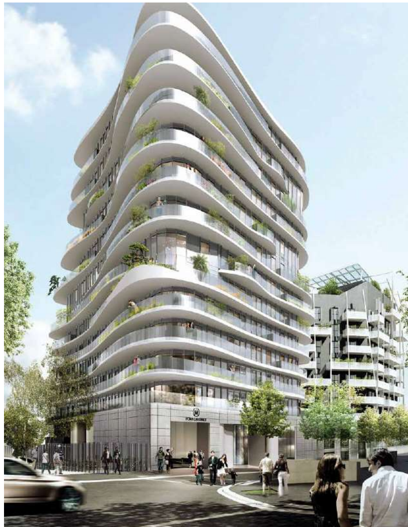
Figure 55 Residential Building. Biecher + MAD. Source: Emerige, 2011.
