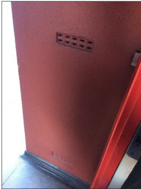
Figure 28: Airing brick on exterior wall.
