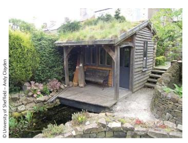
Figure 7.12: Garden building incorporates a veranda, providing an outdoor work or seating space in wet weather. The building is also used to manage rain water which is fed directly into the adjacent pond.
