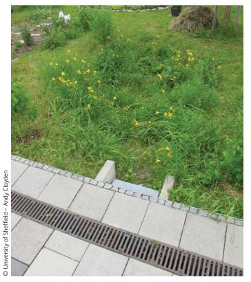
Figure 7.7: A swale is used to gather surface water from the residential area, and allow it to percolate slowly into the main drainage system. This reduction in the rate of surface water run-off allows the main drain systems to better cope with intense rainfall events.
