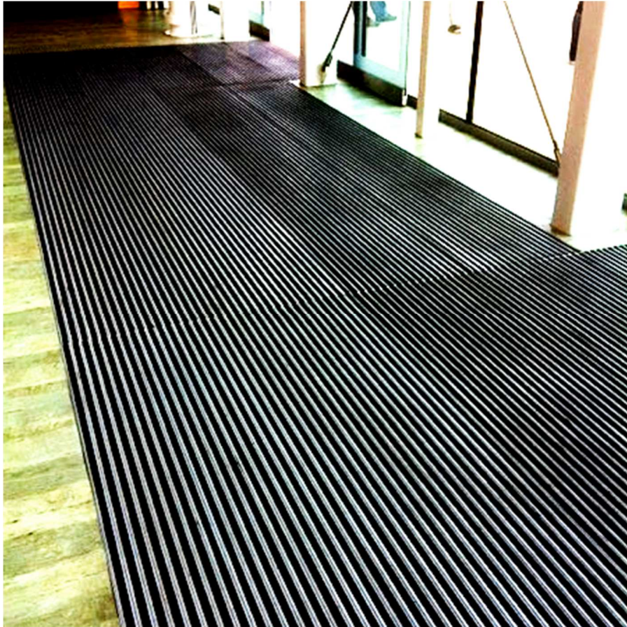
Figure 2. A doormat with high-contrast visual stripes that can trigger epileptic seizures and migraines. (Note that the differences in the physical properties of the two materials forming the stripes are important, but their colour is not. ).
