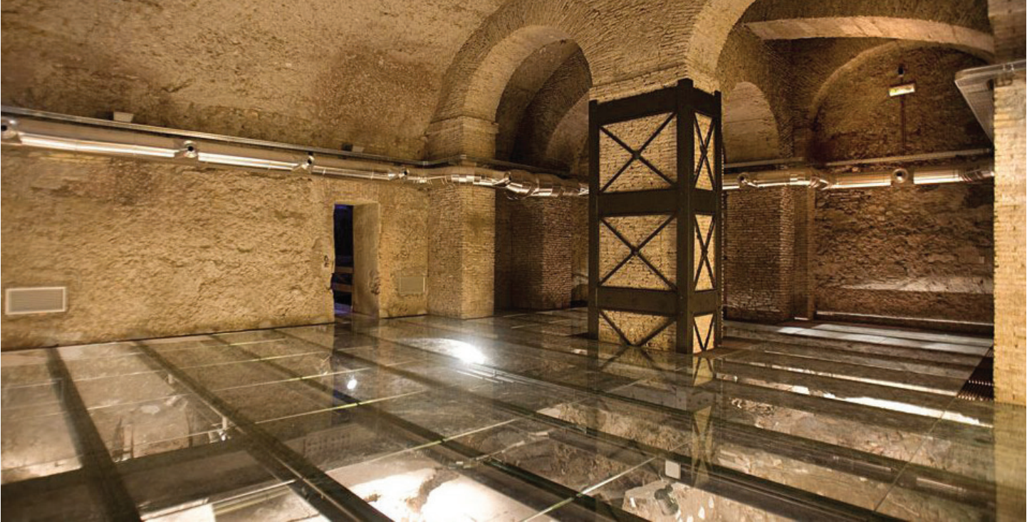
The transparent floor system hovers above the ruins and conceals most of the ASR equipment. Image: Le Domus di Romane Palazzo Valentini Website
