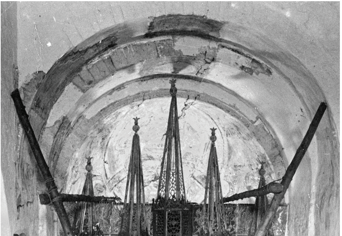
Deep layers of paintings after fresco removal. Photo: Biblioteca de Catalunya, Salvany Archive.
