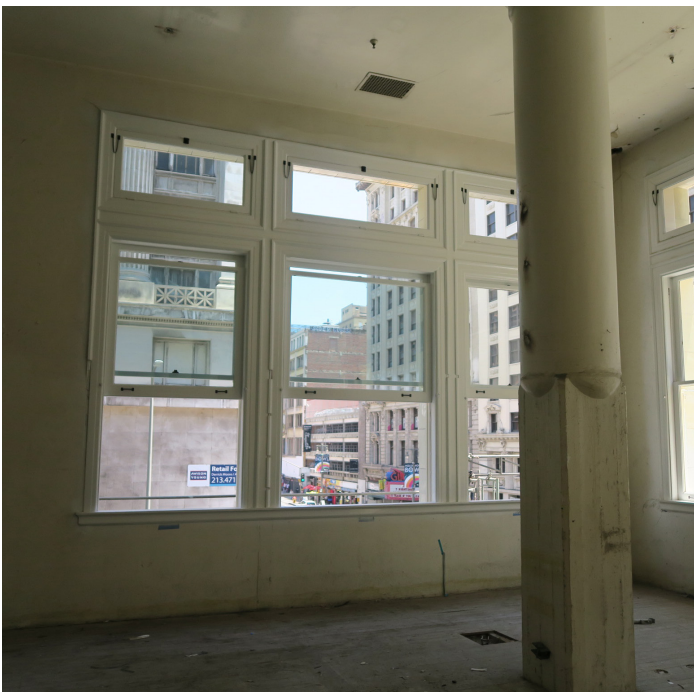
Image [5] Window films that have a slightly blue tint to them were not accepted by the NPS.
