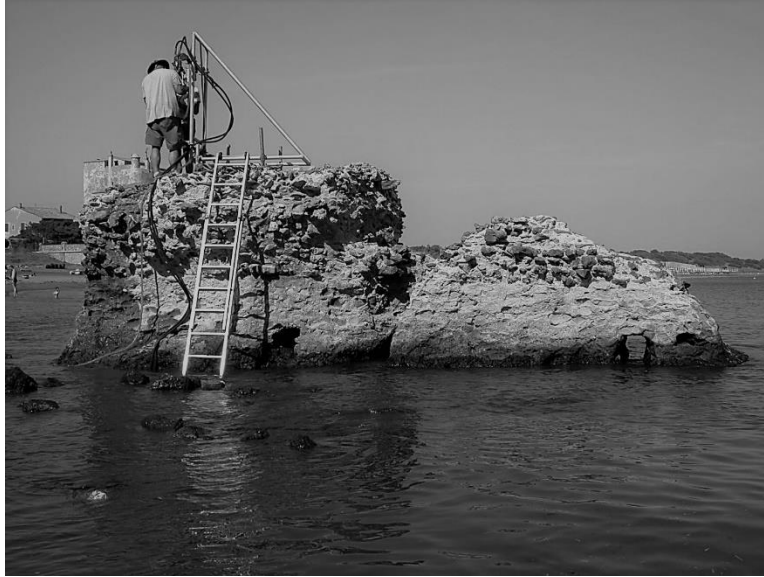
Figure 1. Ancient Roman concrete in marine environment. (PHOTO CREDIT: J. P. Oleson)
