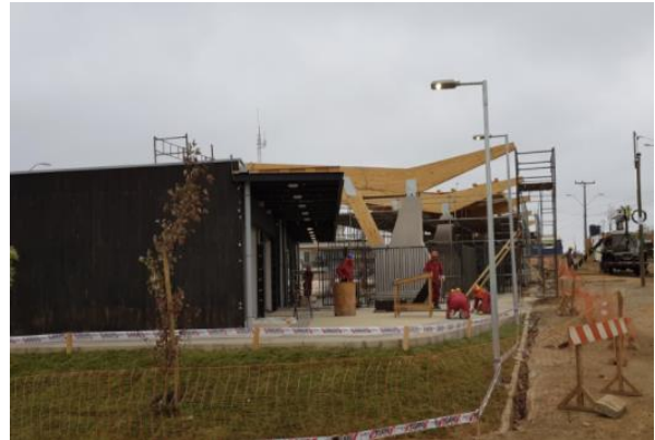
Figure 16 Bus terminal almost completed (March 2018, source: MINVU)
