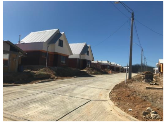
Figure 14 Paved streets and houses almost completed (November 2017)
