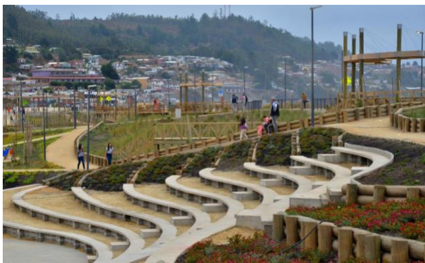
Figure 12 Waterfront park, differences in height will provide protection from future tsunamis or floods.
