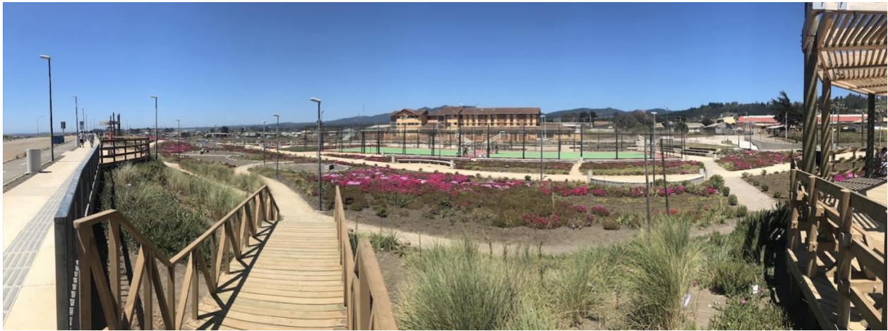
Figure 10 Above: Pellubue post-tsunami, below: Pellubue during November 2017 field trip.
