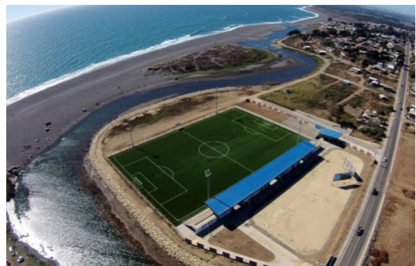
Figure 11 New stadium in Pellubue, built as a resilient infrastructure.
