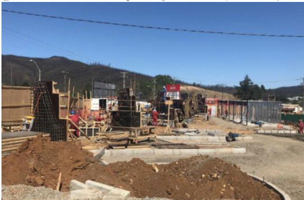
Figure 15 Bus terminal in the process of construction (Nov. 2017)
