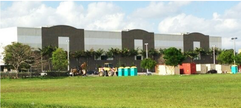
The new press structure
