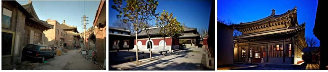
Figure 4.4: Courtyard and Exterior of Dugang Hall, Before and After Restoration
