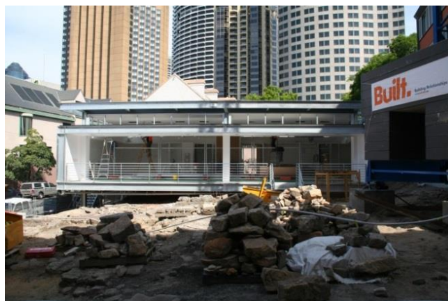
Figure 4.14: The Education Center Being Built, September 2009
