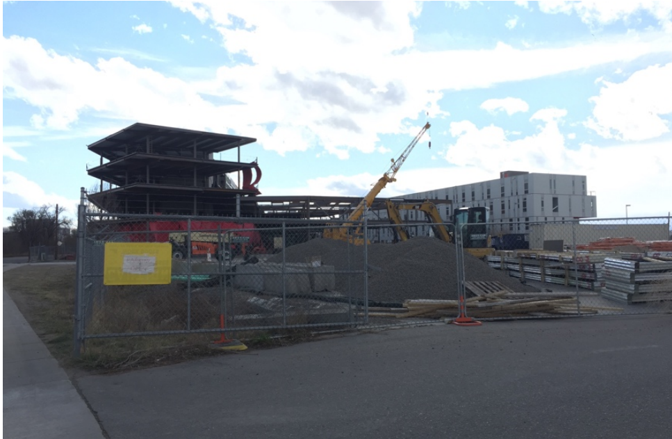
Figure 20: Construction along Ringsby Court (Looking South)
