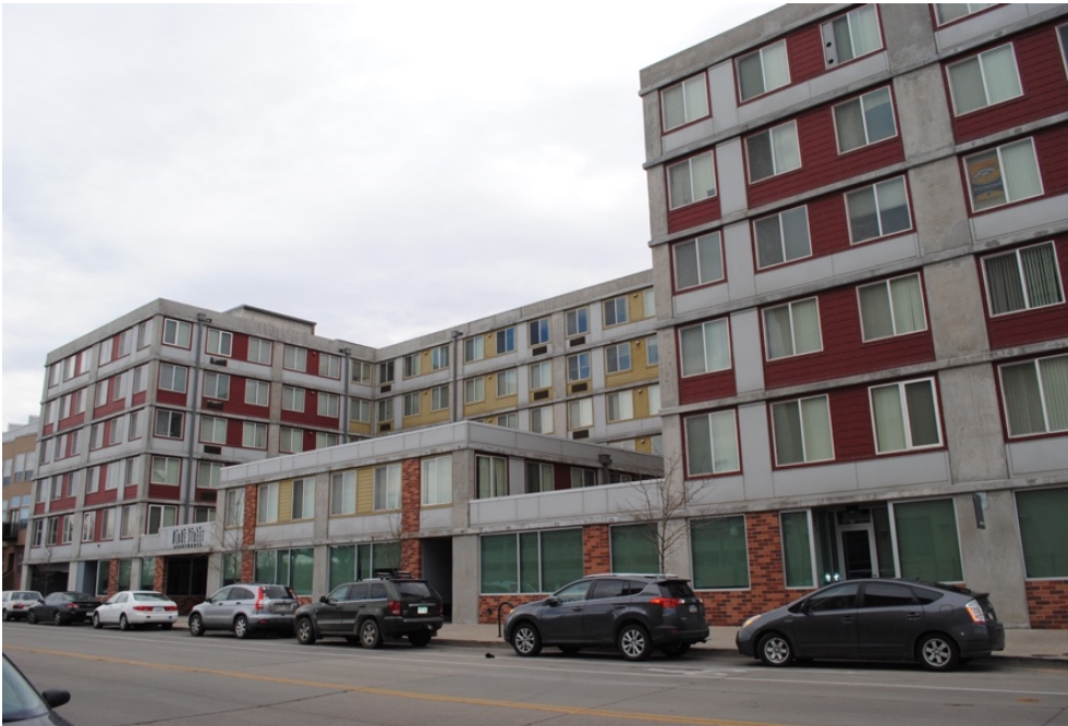
Figure 8: Newer Construction in the RiNo Art District
