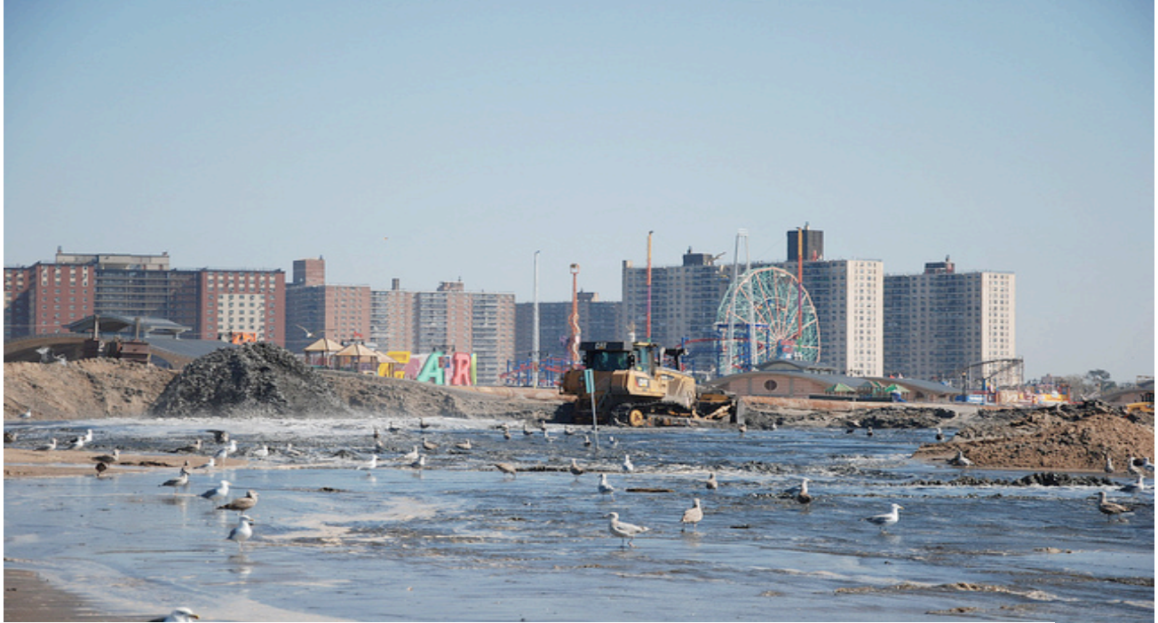
Section 4.1 | Figure 8: Coney Island landmarks are visible as crews work to place sand and restore the beach.
